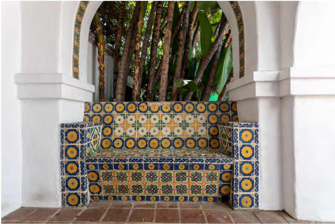
Tiled bench, view looking south.
