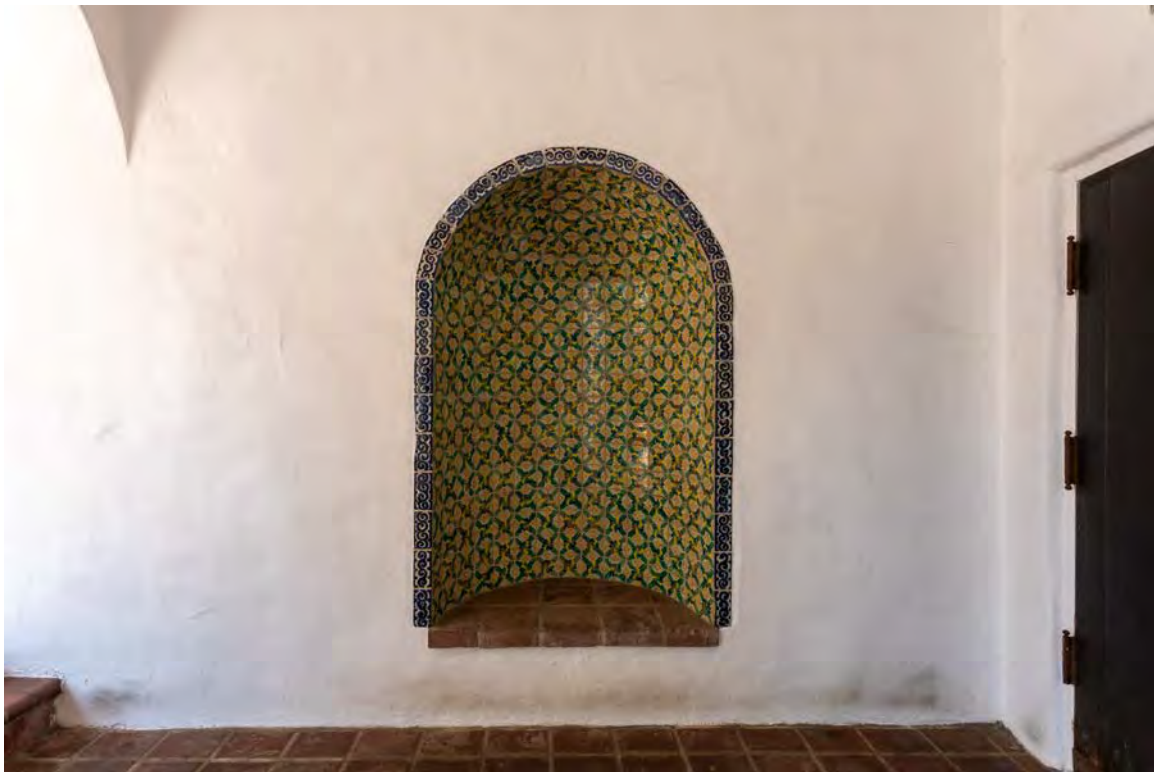
Tiled alcove, view looking north.
