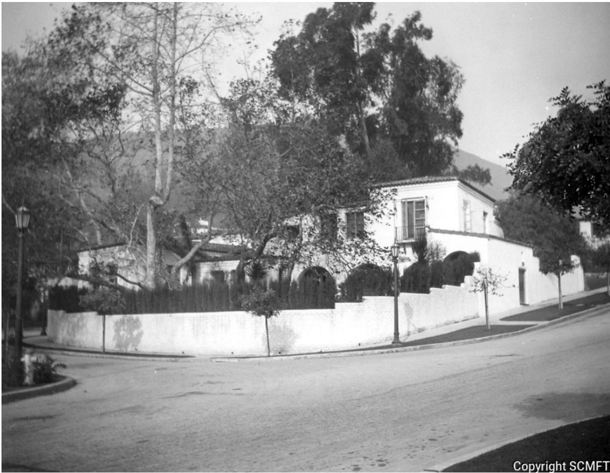
1903 Outpost Drive, view looking northwest across Outpost Drive, circa 1928. HollywoodPhotographs.com.
