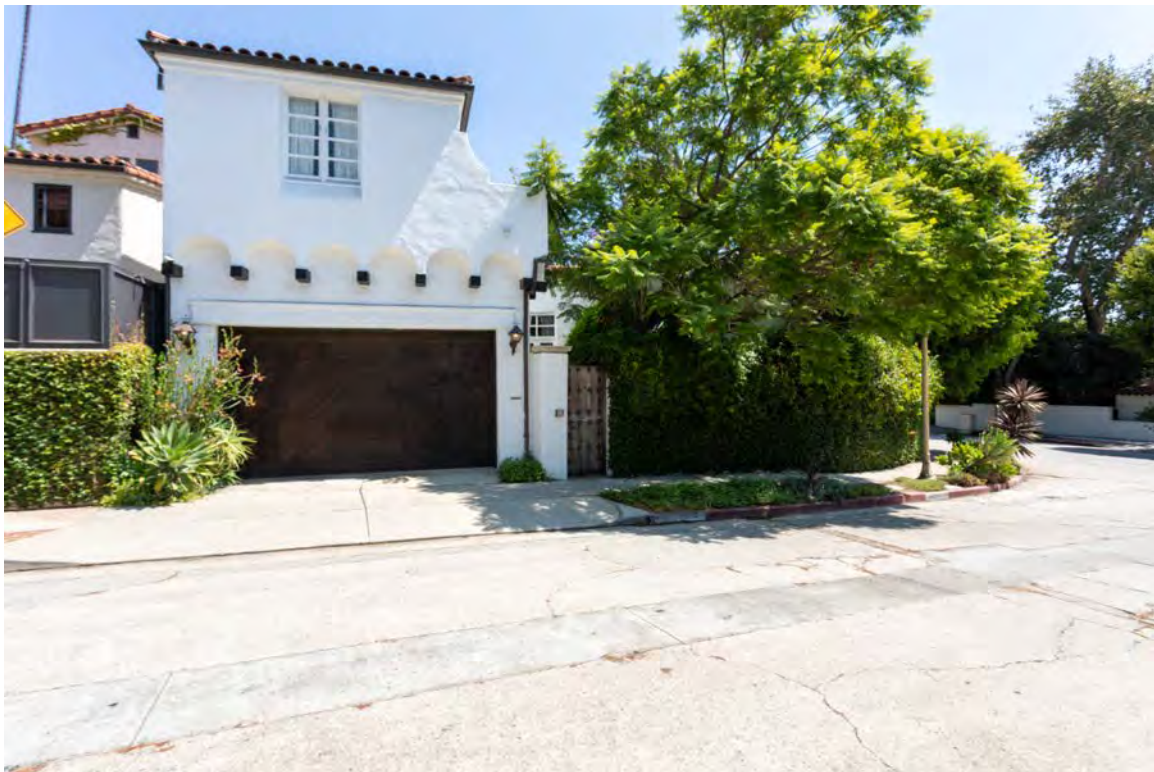
West façade, view looking east.
