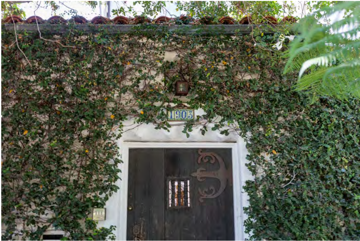
Primary entrance gate detail.
