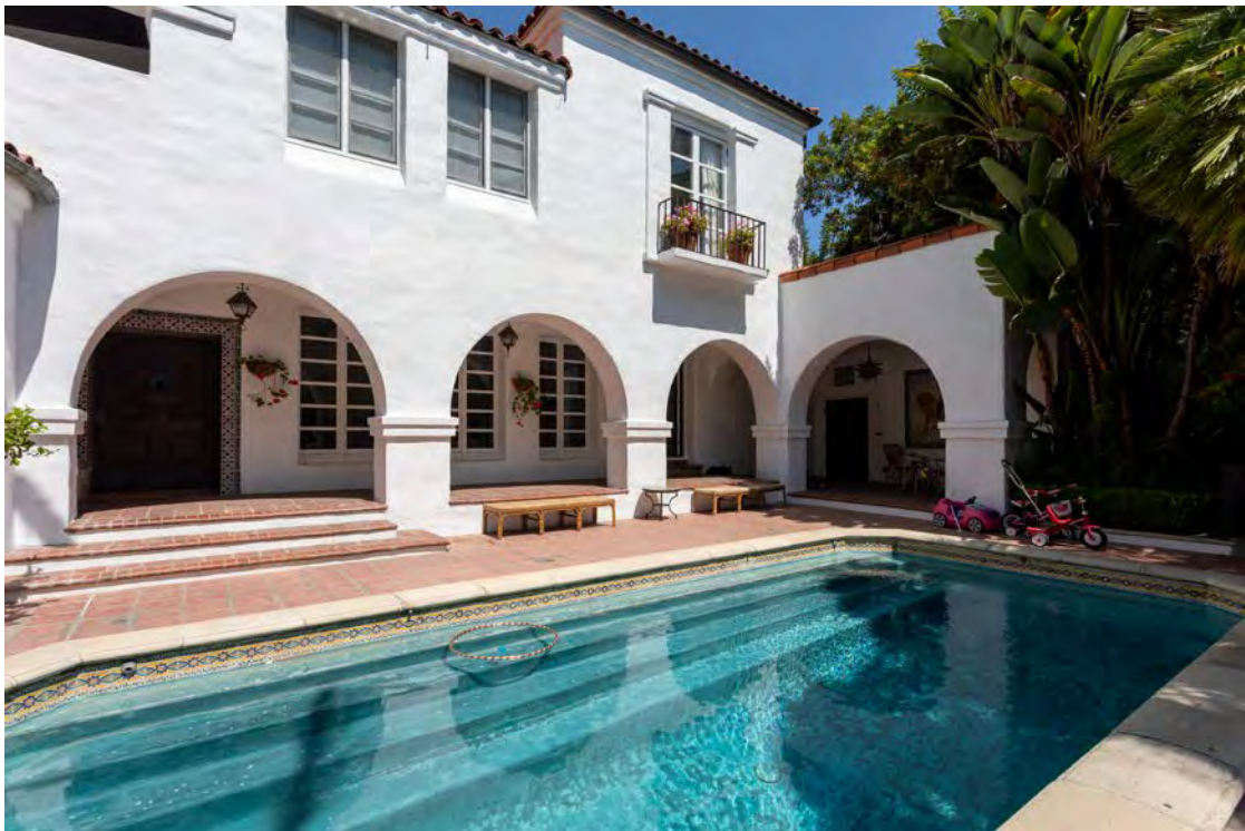
Primary (south) façade, view looking northeast.
