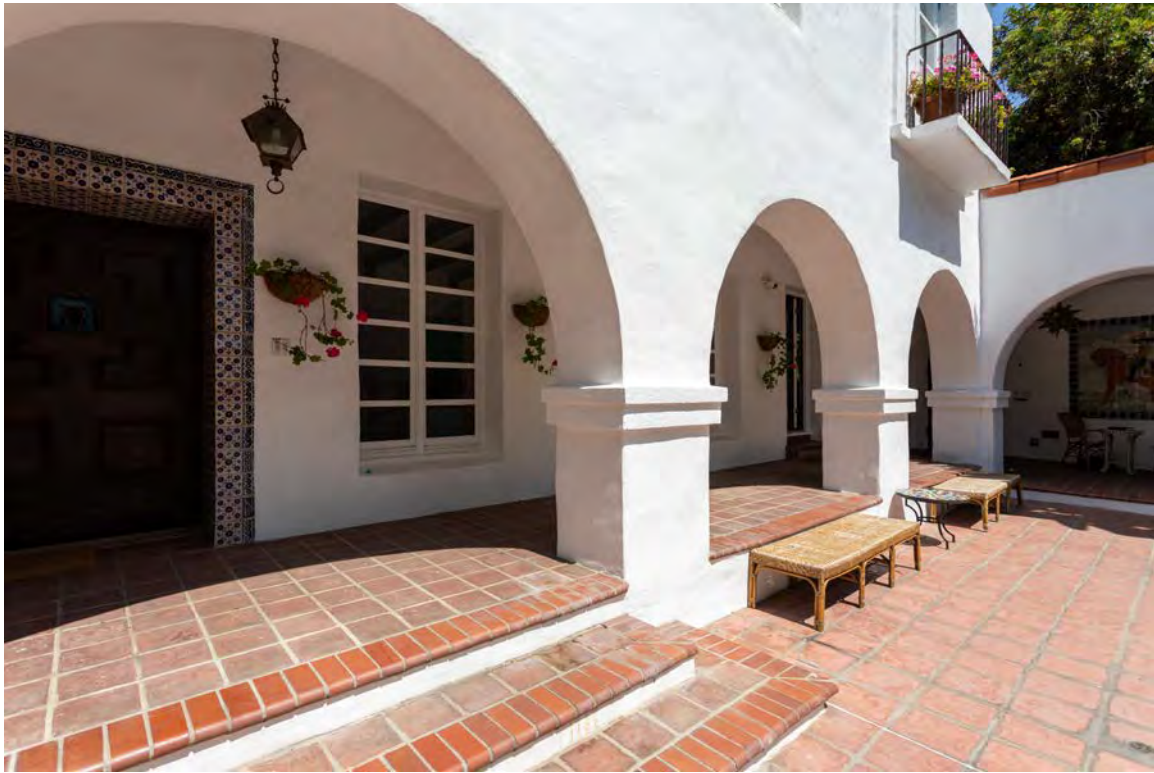
Corredor, view looking northeast.
