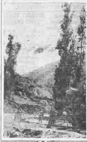
Building Road in Subdivision
