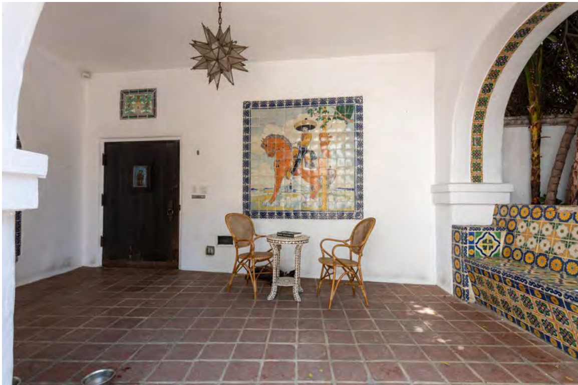
View looking east. The primary entrance gate is visible to the left.
