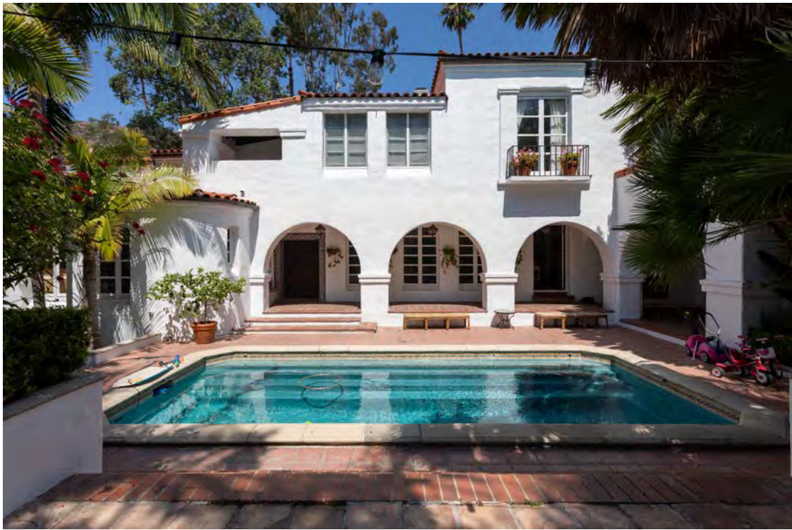
Primary (south) façade, view looking north.
