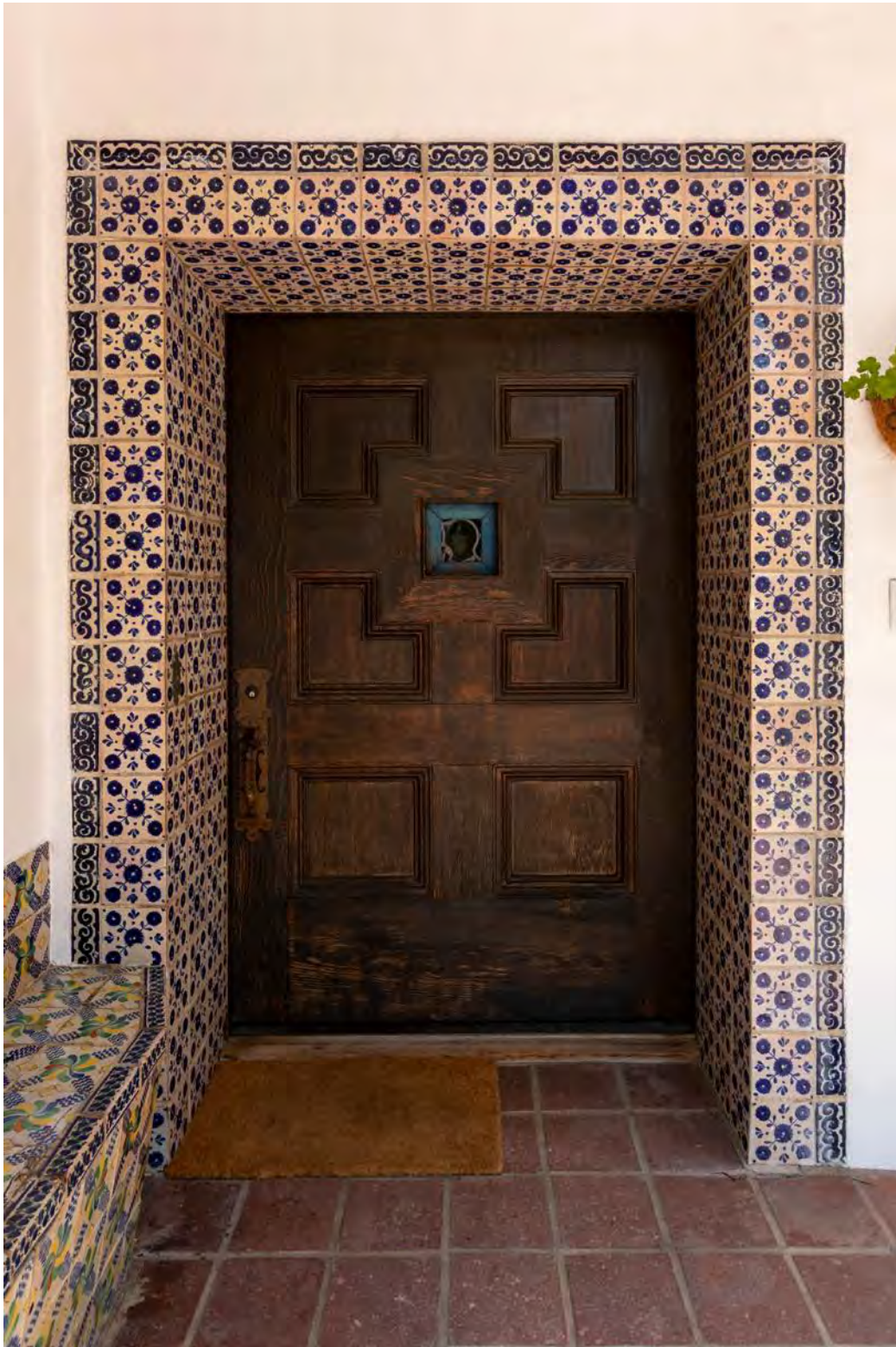
Primary entrance door, view looking north.
